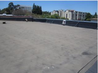
The covering is sloped so that water failing onto the roof is directed to drains in the front and rear corners for the roof (right). Some sediment was noted close to the roof drains: this is indicative of water pooling in these areas. Cracks in the covering were noted throughout the roof (examples below). In addition, there were sever examples of lifted and/or poorly sealed seams at sheet edges.
