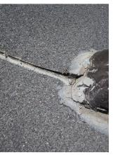
Trim at the NW edge of the upper roof was rotten (right).
