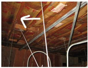
A plastic-lined box was located between the suspended ceiling at the underside of the roof this is excellent evidence that the roof leaks in under wet conditions. What may be additional water damage was noted at the base of the exterior wall in the rear of the unit (right).
