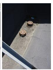
The condition was also similar with cracks in the covering and lifted and/or poorly sealed seams evident throughout the upper roof.
