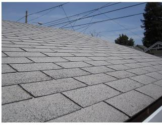
Curled shingles were present throughout the roof and at the edges of the roof. The right side of the roof at the rear was covered with moss. Flashings at roof vents are rusted, and have been repaired with roofing cement a number of times.
