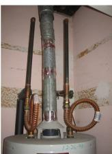
valve. This is an important safety device and should not be tampered with. The T/P relief valve appears to be properly installed. Piping from the valve is routed to the exterior. The exit pipe is an important safety feature, which should not be moved or blocked off.
